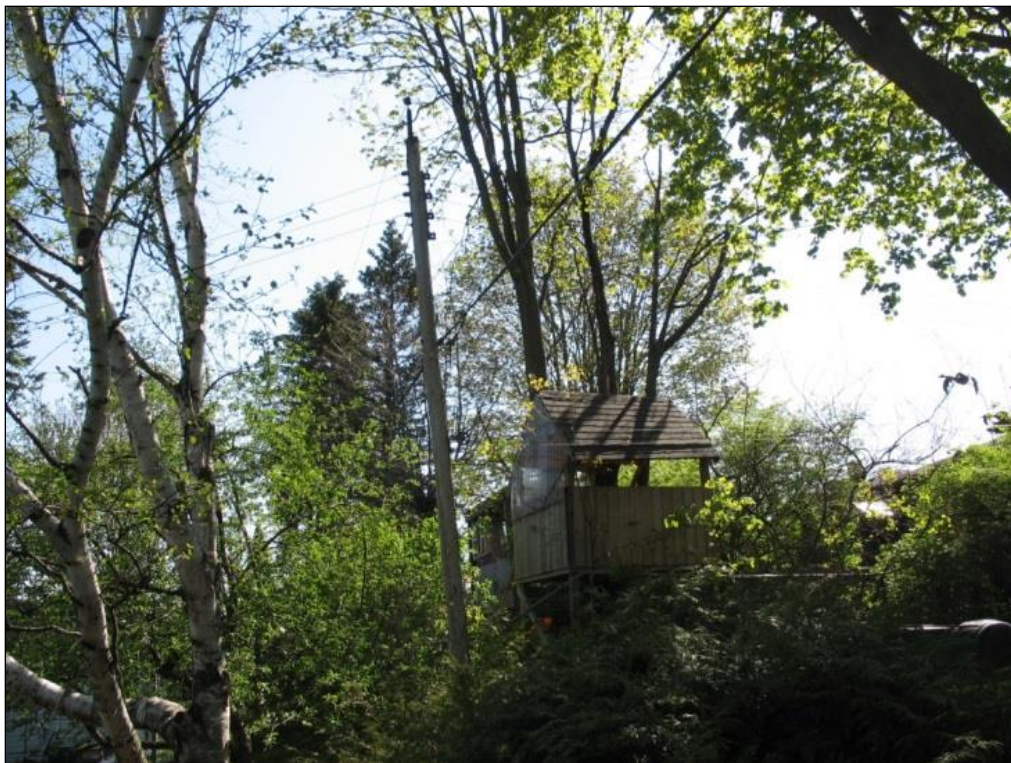
13 Figure A07 - 1: Tree-house Close to Pole and Energized Conductor
