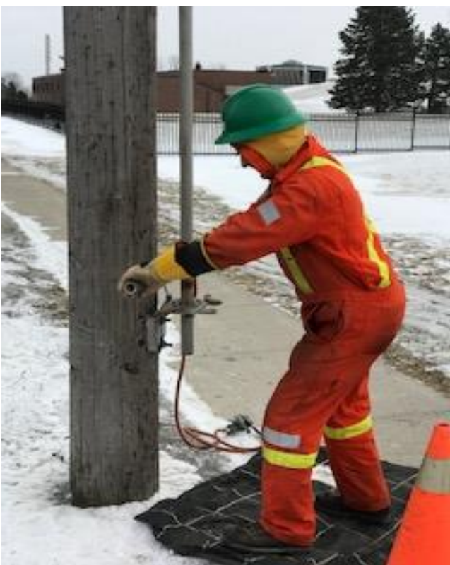
Figure A11 - 1: Manual Load Break Operation
