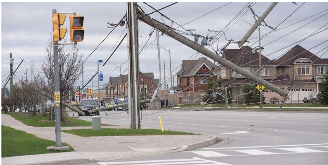
Figure A05 - 10: High winds caused down power lines on Bayview Avenue in 2018.
