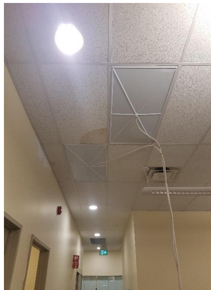
Figure A17 - 2: Water Damage Nebo Road Roof
