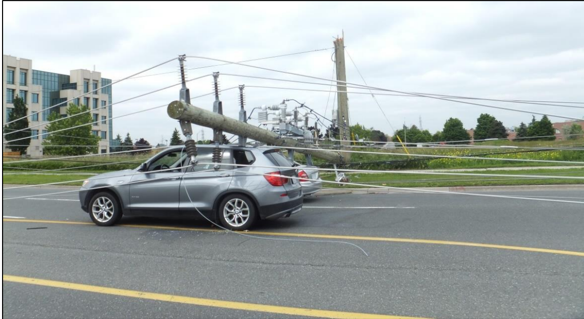
Figure 5.3.3 - 19: Failure of Legacy Wood Pole on Islington Avenue in Vaughan on October 15th, 2017
