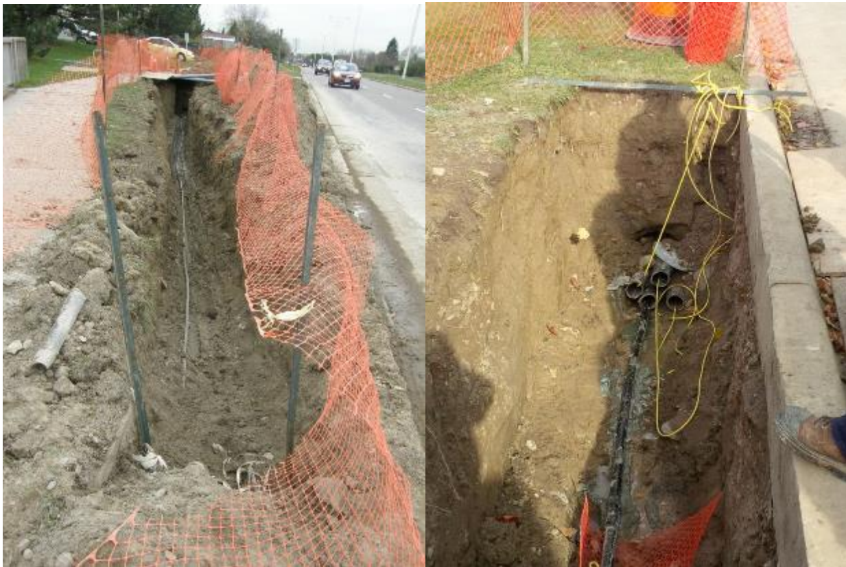
9 Figure A10 - 4: Underground Cable Replacement
