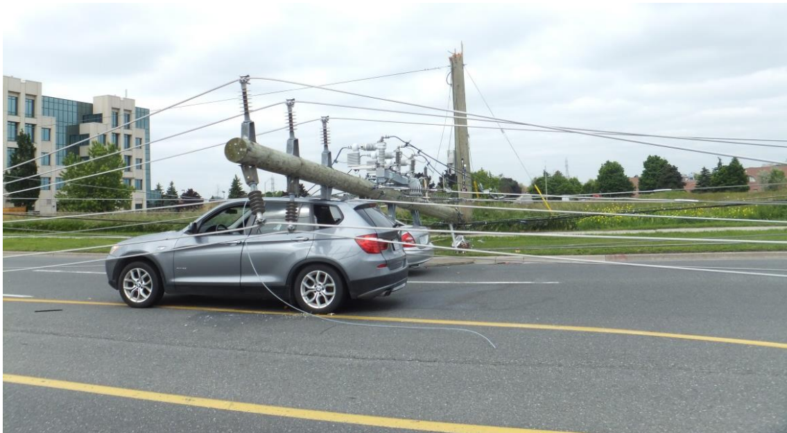
6 Figure A05 - 8: Failure of Legacy Wood Pole on July 17th, 2014
