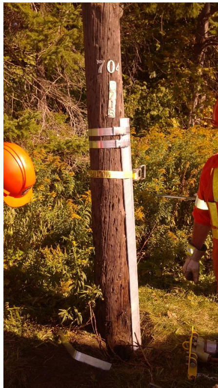
14 Figure A05 - 3: Wood pole reinforcement process and final outcome
