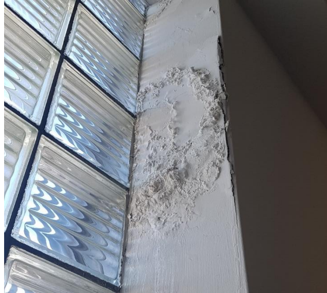
Figure A17 - 2: Water Damage Nebo Road Roof
