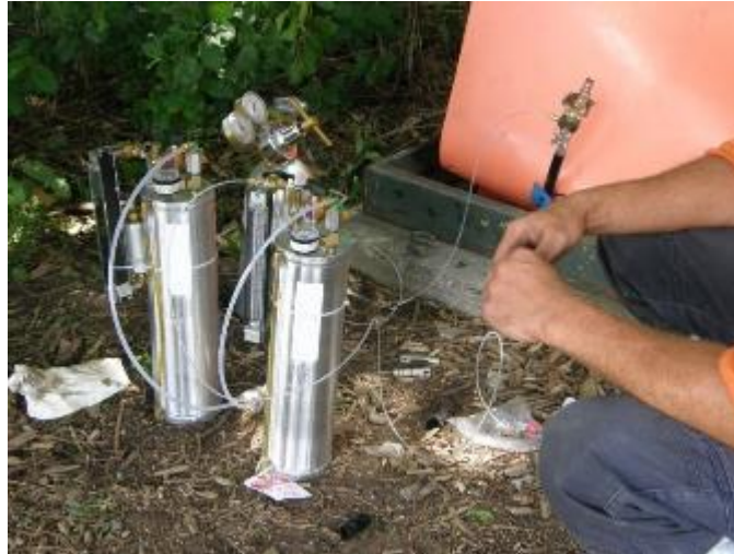
4 Figure A10 - 3: Underground Cable Rehabilitation by Cable Injection
